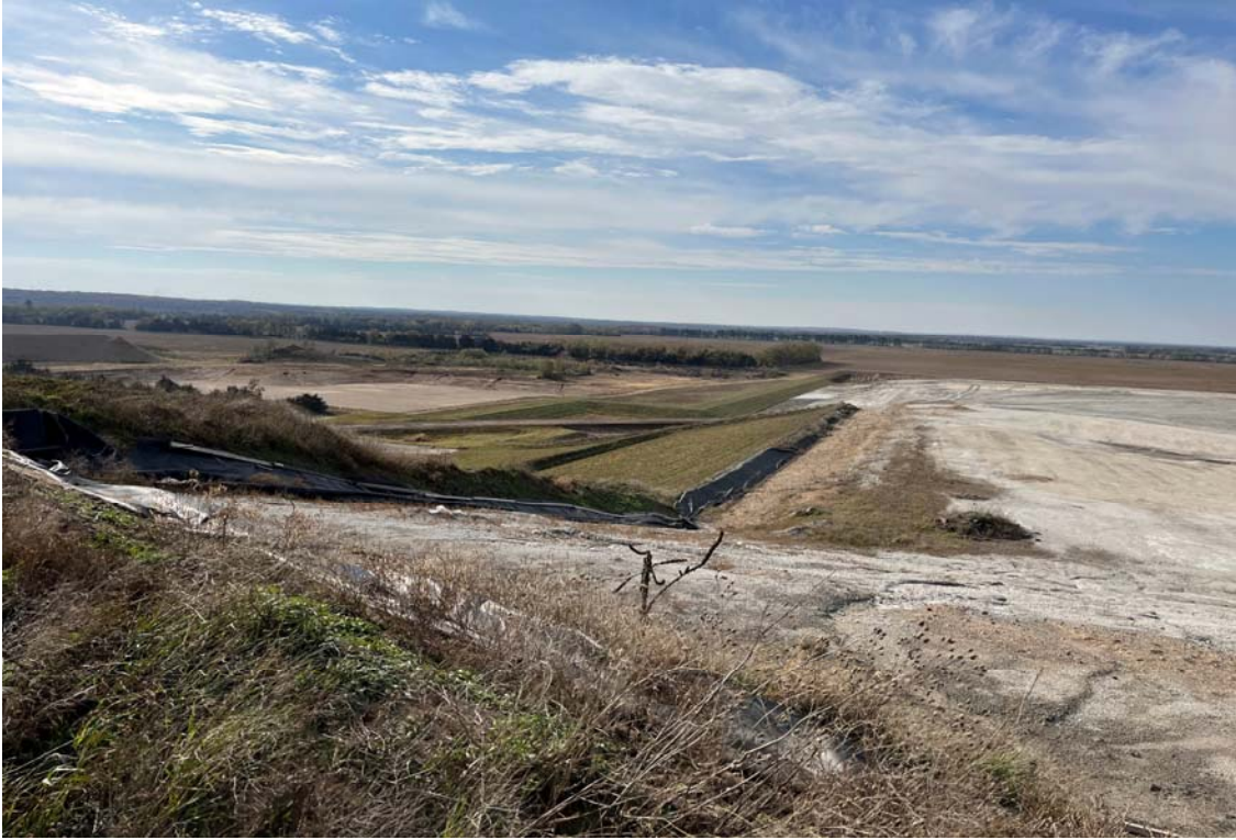
Photo 7 Run-off control berm installed on all final cover terminations, looking west. 11/5/2021
