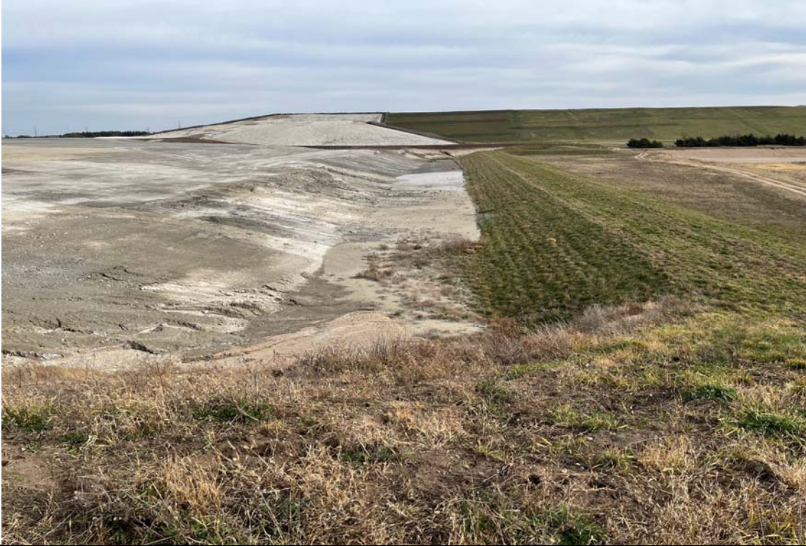
Photo 5 South embankment, looking east. 11/5/2021
