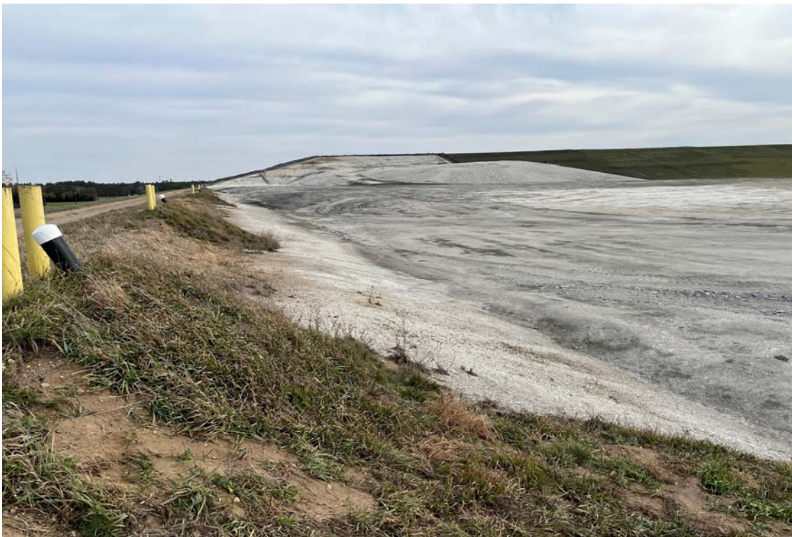
Photo 2 Interior of north embankment, looking east. 11/5/2021
