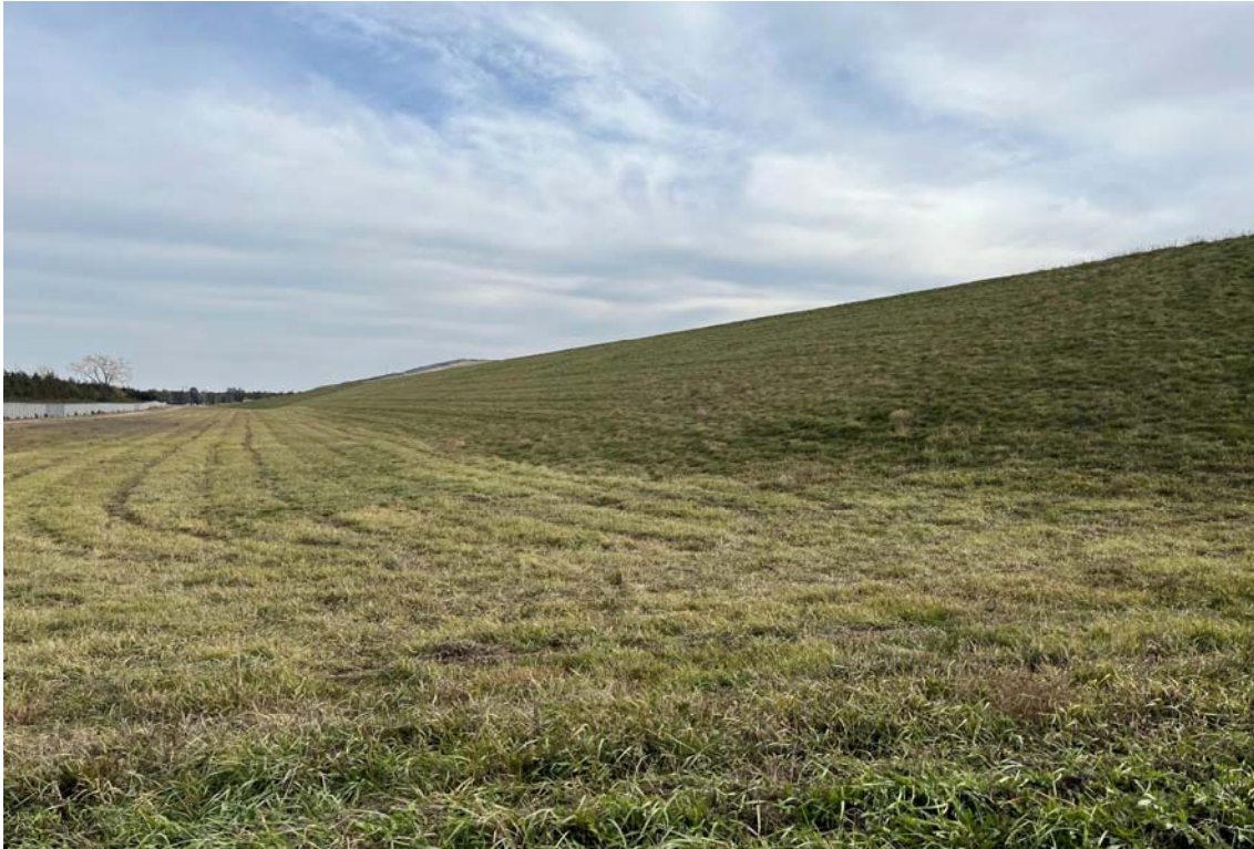
Photo 1 Exterior of north embankment, looking east. 11/5/2021
